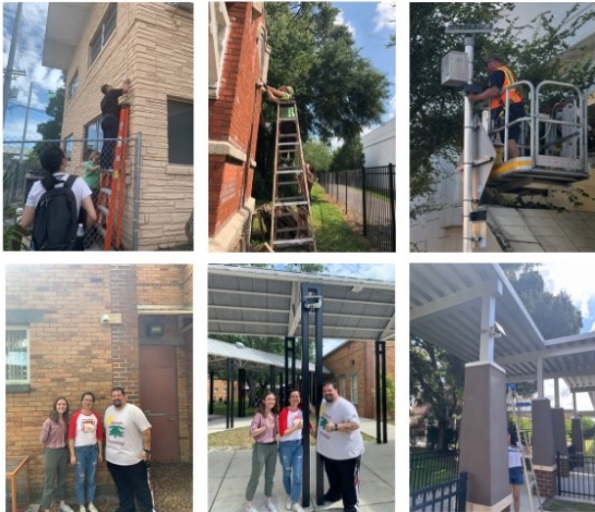
Figure 12. Installations at community sites. The top row, from left to right, shows installations at the New Mount Zion Baptist Church, Tampa Heights Junior Civic Association, and on a Rectangular Rapid Flashing Beacon post along the Tampa Heights trail. The bottom row shows installations, from left to right, at Seminole Elementary School (the left image is the PurpleAir II, and the center image is the Clarity Node-S), and Robert J. Saunders Sr. Public Library.
