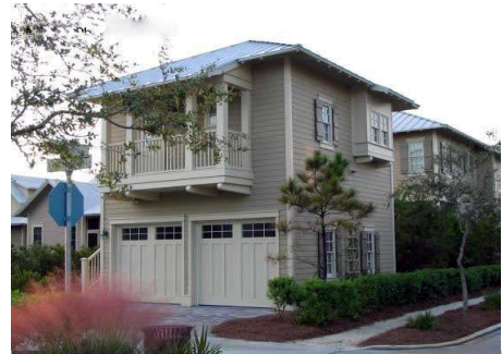
Accessory units similar to the one pictured are encouraged within traditional neighborhood developments.
