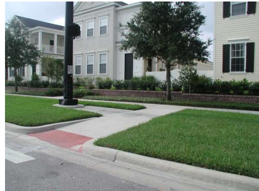
The texture and color contrast before the crosswalk is used to warn pedestrians that they are entering a vehicular area.
