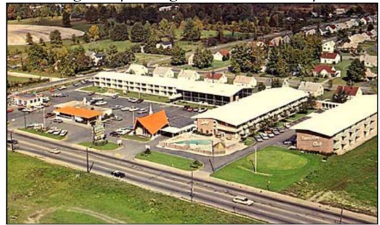
This type of access management, where one business has multiple non-connecting parking lots, is not recommended.
