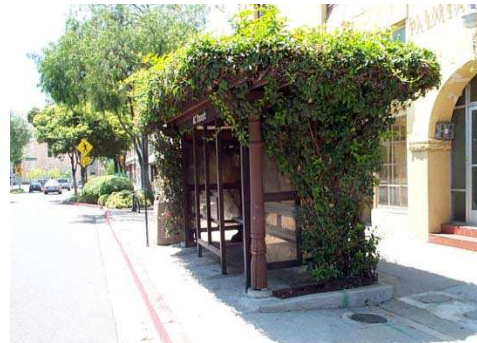
Poorly maintained landscape obstructs views to and from this shelter.
