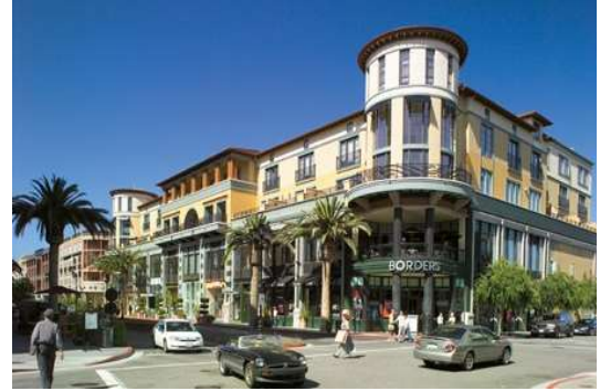
This large building mass is broken down with variation of height, setbacks, and architectural treatments
