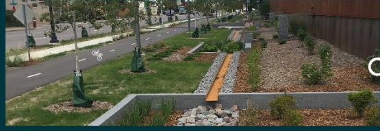
Complete Street Features & Enhanced Stormwater Facilities
