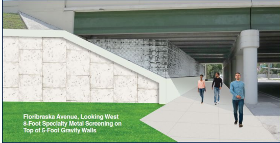
Floribraska Avenue, Looking West 5-Foot Fencing on Top of 8-Foot Gravity Walls
