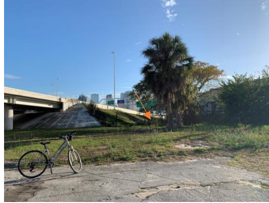
At Henderson Ave looking south.
