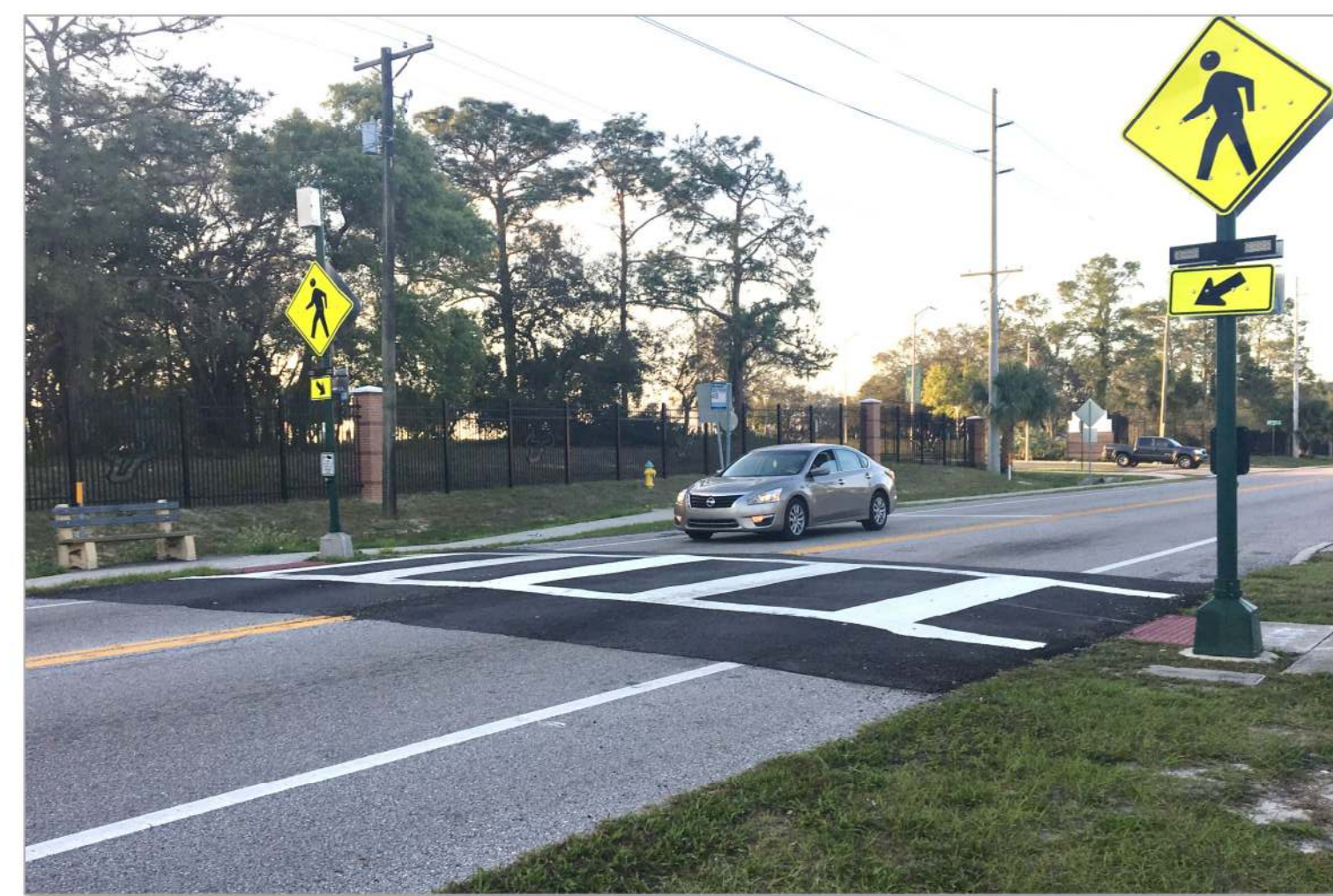
50 th Street – Raised Crossing
