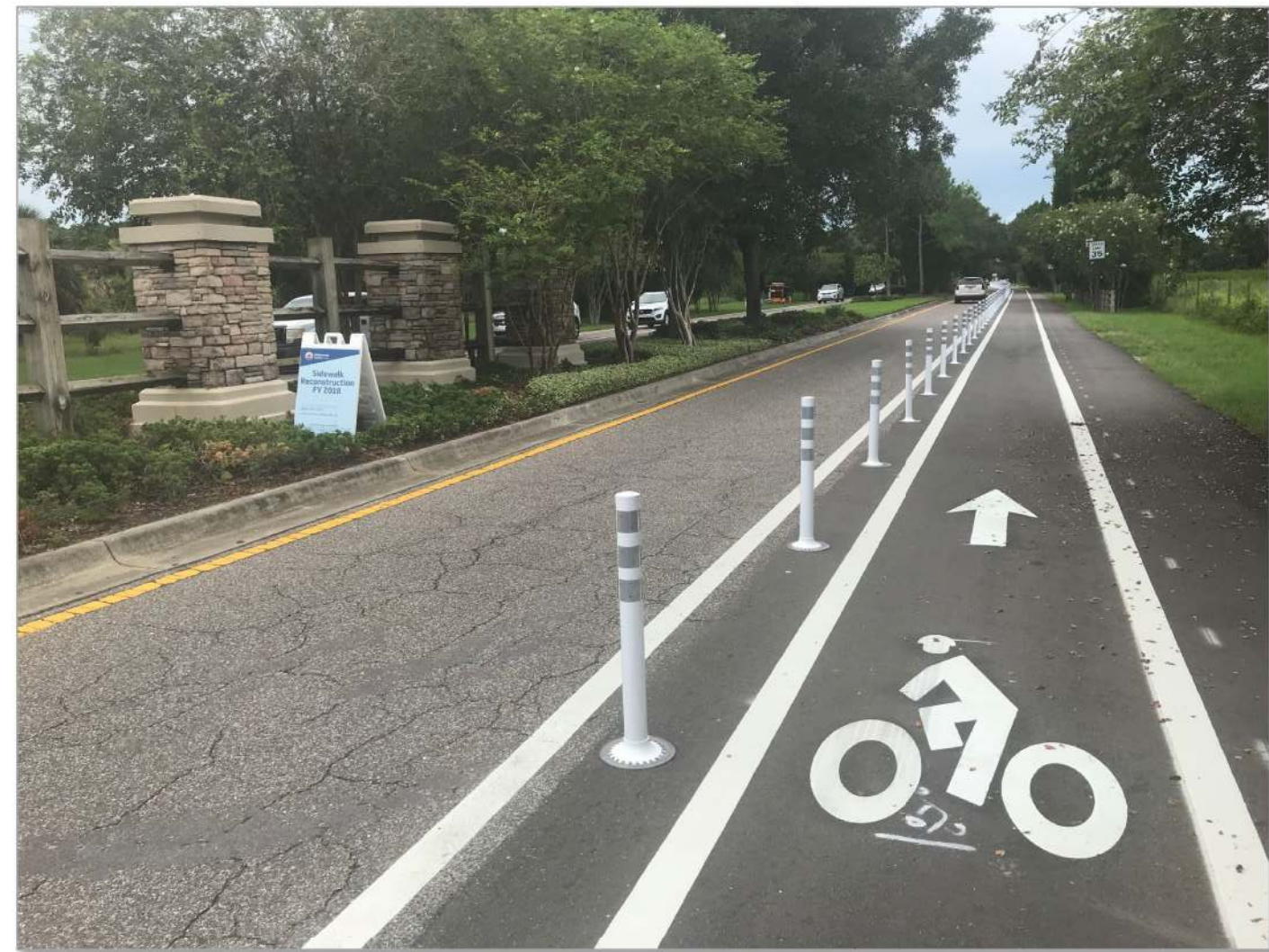
Covington Garden Drive – Bike Lane Delineators
