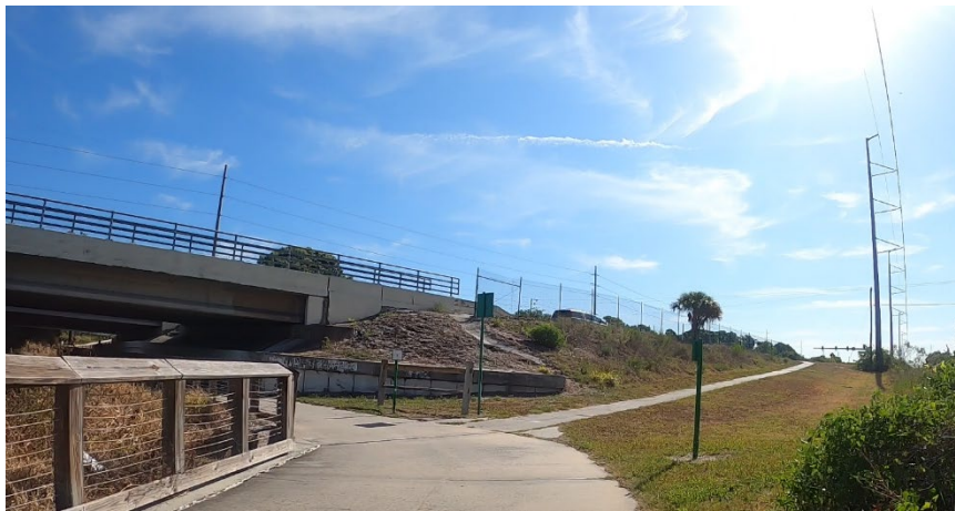
Connection to Linebaugh Avenue
