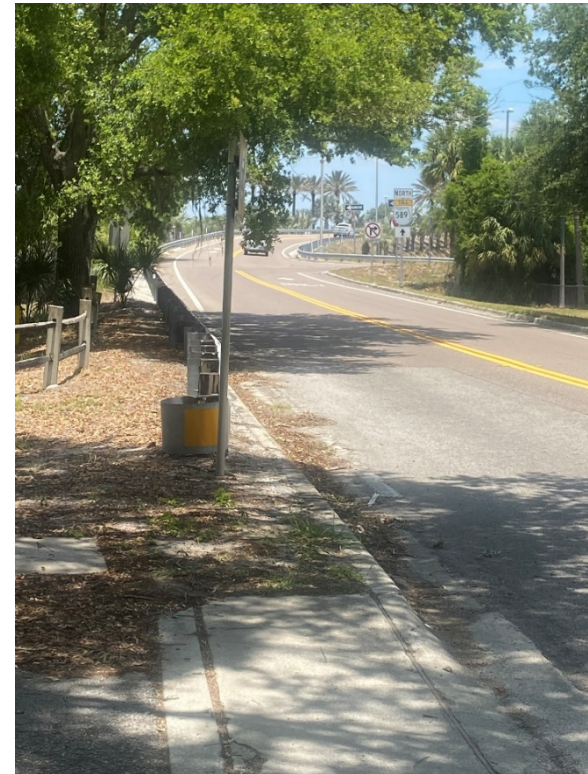
Trailhead Entrance on Wilsky Boulevard; Veterans Expressway Ramps in Distance
