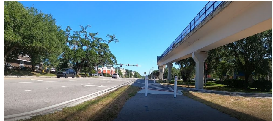
Driveway Crossings and Pedestrian Bridge – Gunn Highway/Citrus Park Drive
