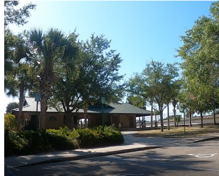
Channel Park Trailhead Amenities
