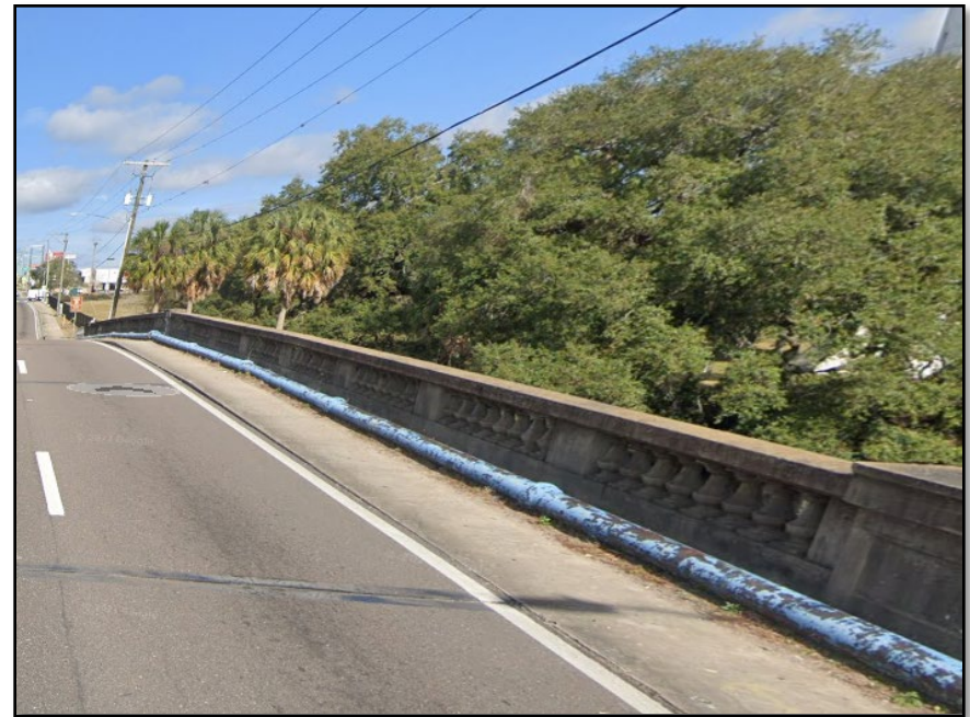
Sidewalk on N Florida Avenue over Hillsborough River
