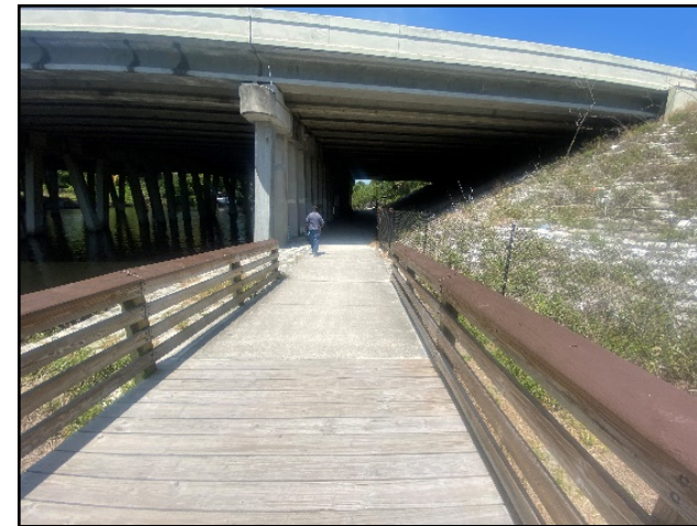
Boardwalk Under I-275
