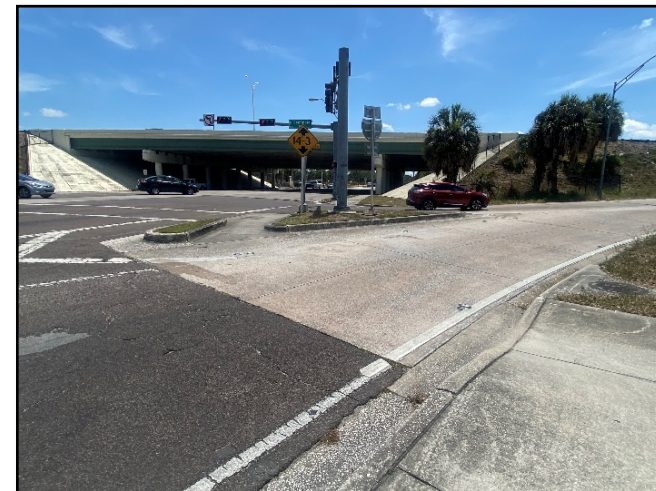
Pedestrian Crossing at E Bird Street / I-275 Southbound On-Ramp
