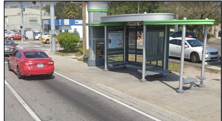
MetroRapid Stop Along N Nebraska Avenue at Waters Avenue
