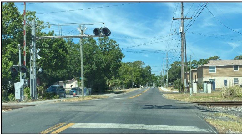
Pedestrian Crossing over Railroad Tracks Railroad Crossing
