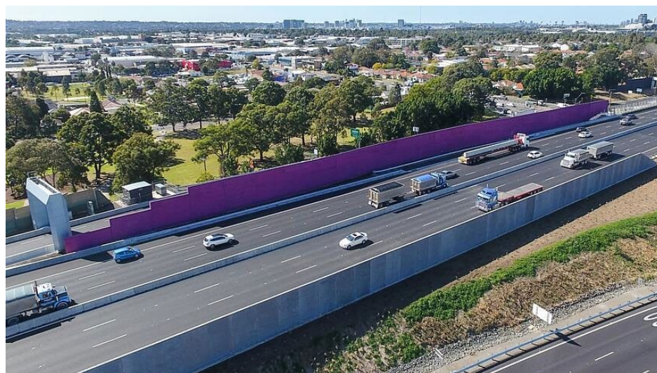
Figure 7: A Hebel sound barrier of autoclaved aerated concrete mounted on a highway overpass. (Source: Hebel)
