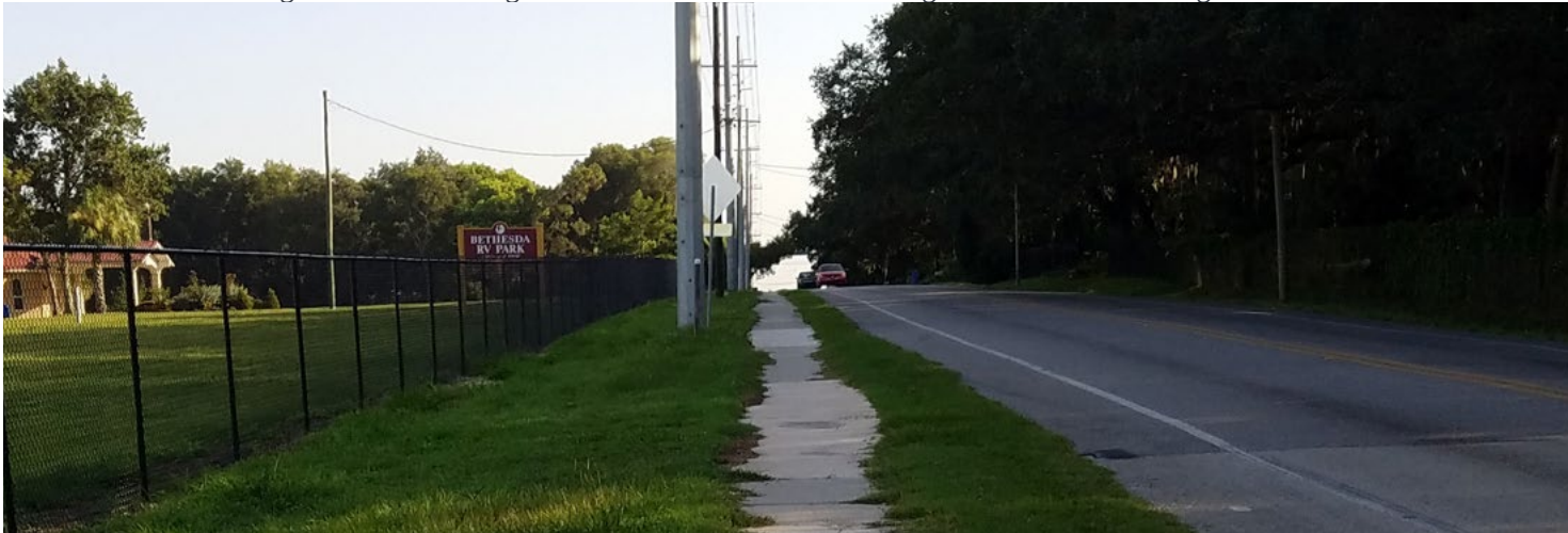
Figure 32 - Existing Conditions at Old Hillsborough Avenue and Mango Road
