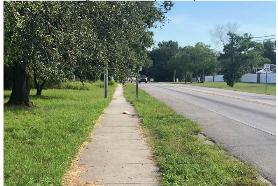
Figure 2 - Sidewalk (West Side)
