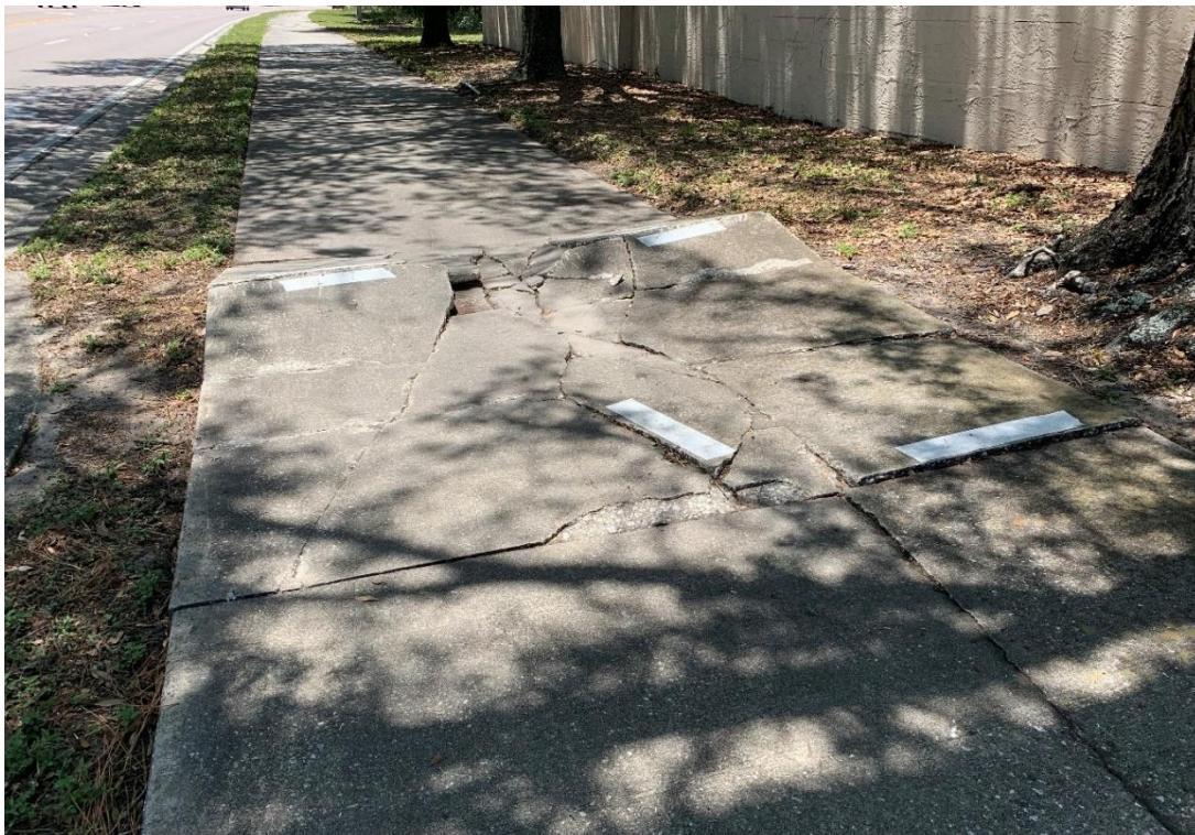
Fletcher Avenue, east of Armenia Avenue, looking east
