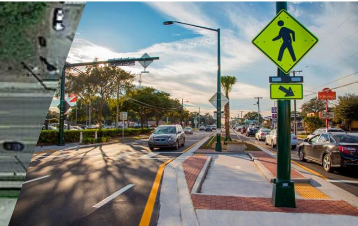
Added Ped Refuge Islands & Mid-Block Crosswalks
