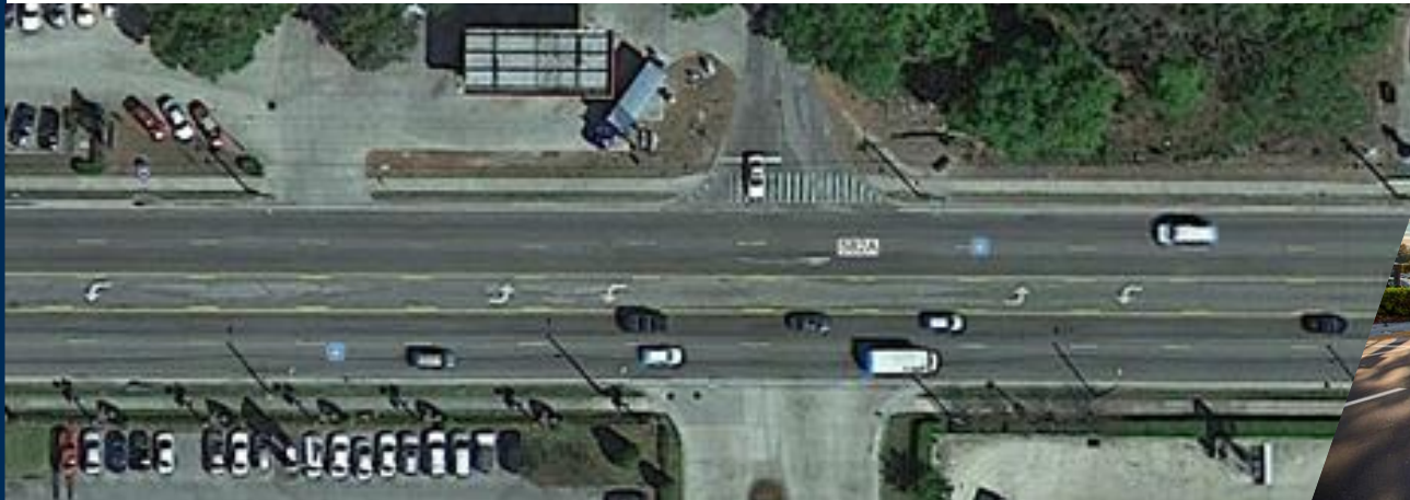
Replaced Two-Way Left Turn Lanes (TWLFL)
