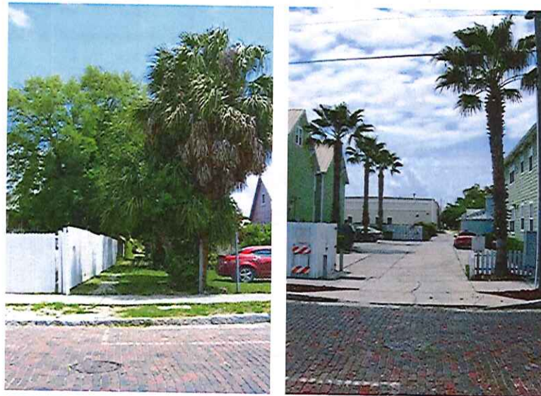
As shown in the above images showing alley conditions from adjoining blocks between 4 th and 5 th Avenues, the alley network in Ybor CRA 2 is uncomplete.
