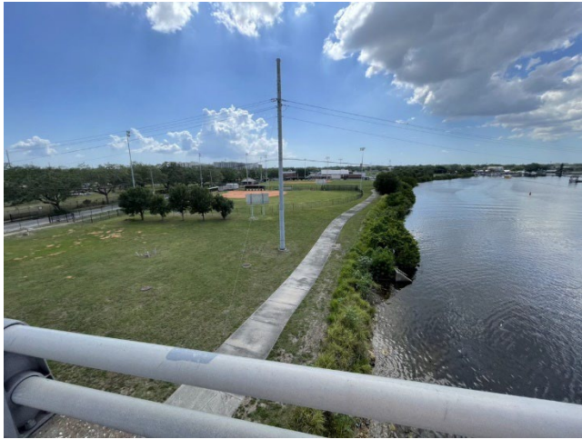
Image 57: Shared Use Path Along River Behind Schools (will be incorporated into extension of Riverwalk)
