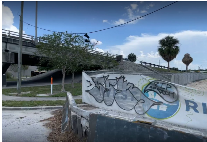
Image 67: Debris Blocking Access to Pedestrian Path
