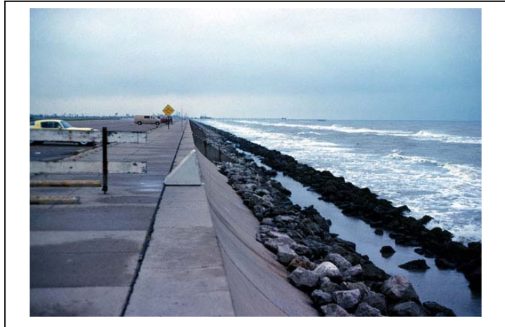
Figure 3-5 Example of seawall for coastal defense combined with a revetment in front to dissipate wave energy.
