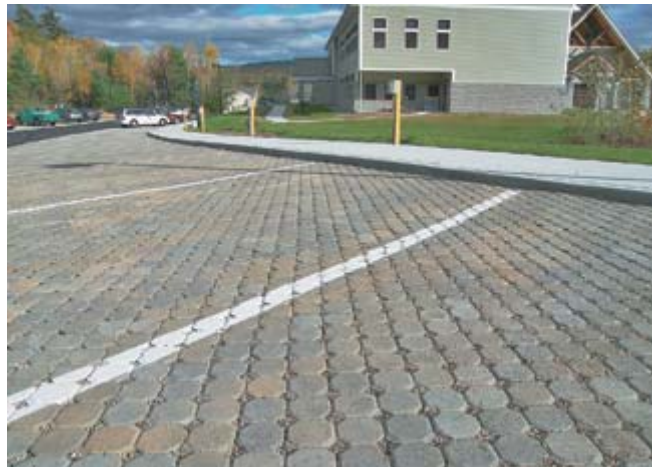
Figure 3-23 Installation of permeable pavers in a parking area to enhance drainage in a large space.
