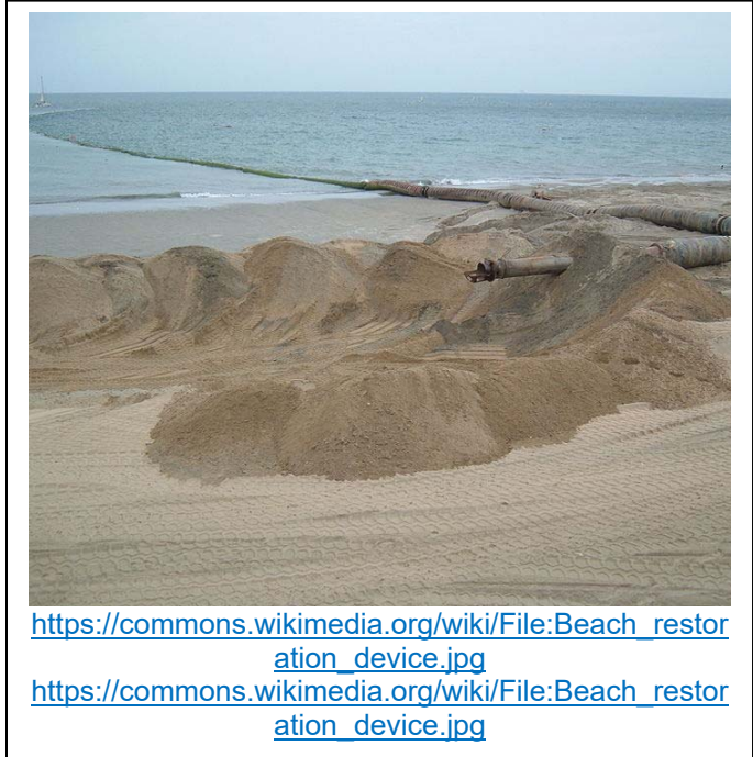
Figure 3-2 Beach nourishment process. Sand is being deposited on the beach from dredging operations offshore.
