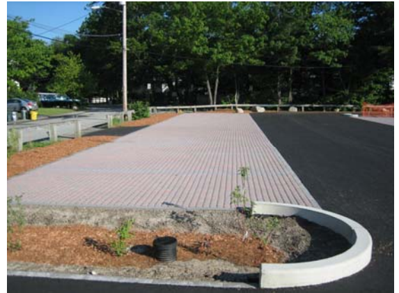
Typical green parking area with integrated planting areas and permeable pavers as per Massachusetts Executive Office of Energy and Environmental Affairs.
