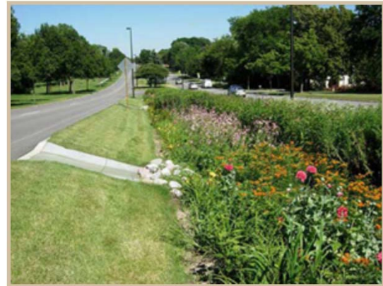
Typical bioswale with directed drainage from roadway as per Soil Science Society.
