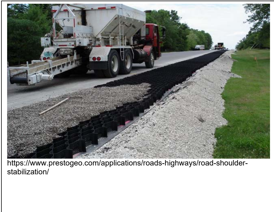
Figure 3-21 Installation of soil mats on a shoulder to reduce erosion and protect the road base against damage from water flow events.
