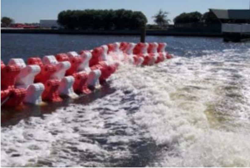
Figure 3-8 Floating wave attenuation device 17
