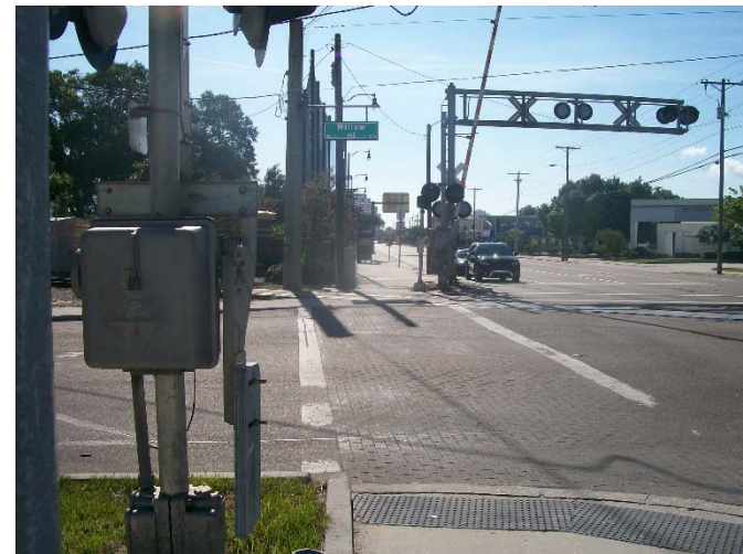
Figure 40: Missing Pedestrian Signal, Kennedy Blvd at Willow Ave, Looking East
