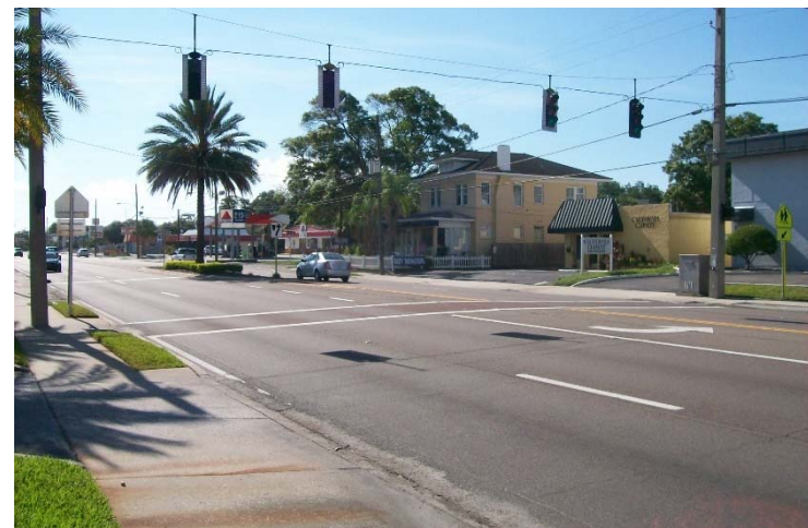
Figure 34: Existing Mid-Block Crossing, Kennedy Blvd between Gomez Ave and Bungalow Park Ave, Looking Southeast
