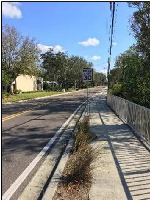
Figure 2.1 Mendonsa Road sidewalk. Source: Project Team.
