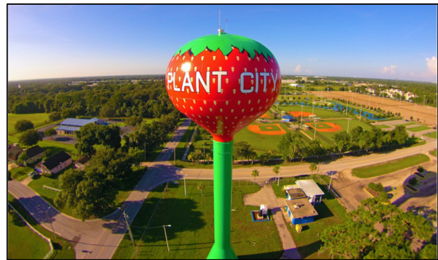
Plant City Water Tower. Source: Plant City Observer.
