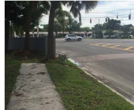
Bay Crest Community sign blocks access to sidewalk at Lopez Drive and Memorial Highway
