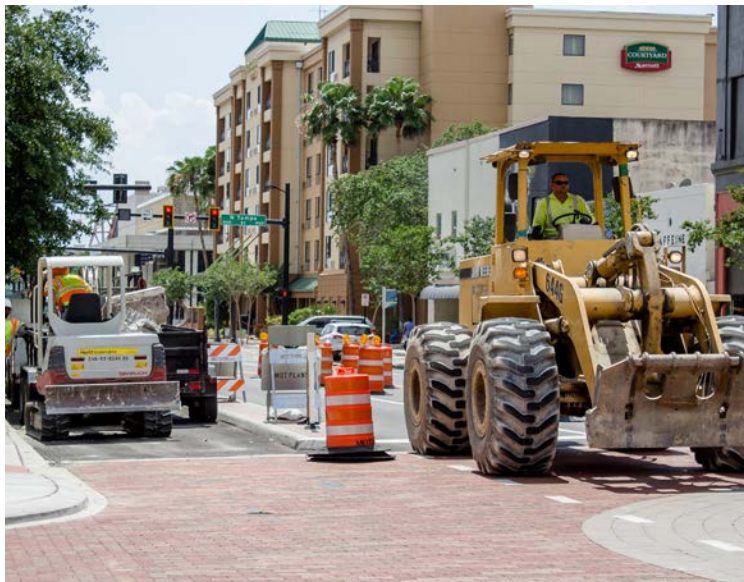
Road reconstruction on East Cass Street in Downtown Tampa
