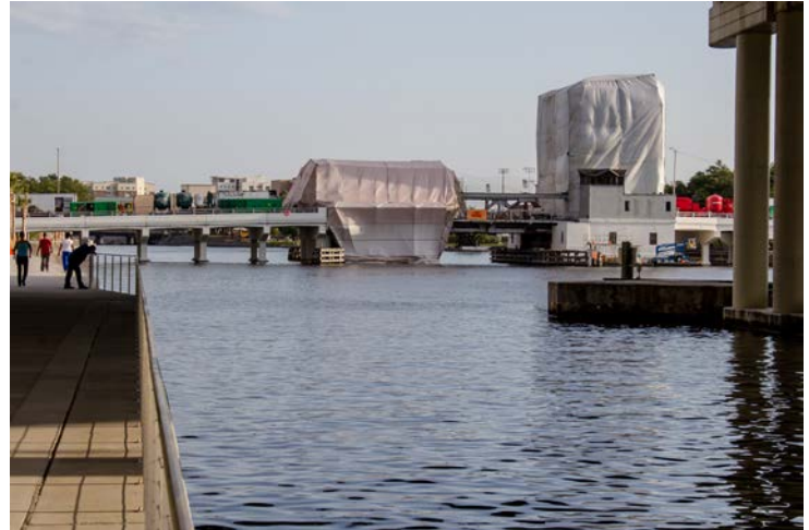
Bridge reconstruction, West Laurel Street and Hillsborough River
