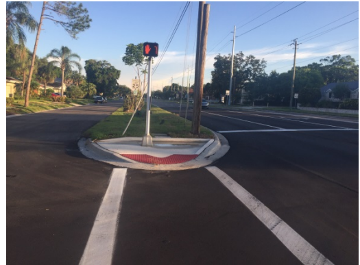
New Intersection improvements at Lopez Drive and Memorial Highway
