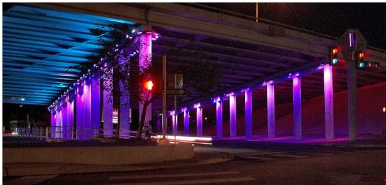
Figure 7. Example of underbridge lighting color wash on columns.
