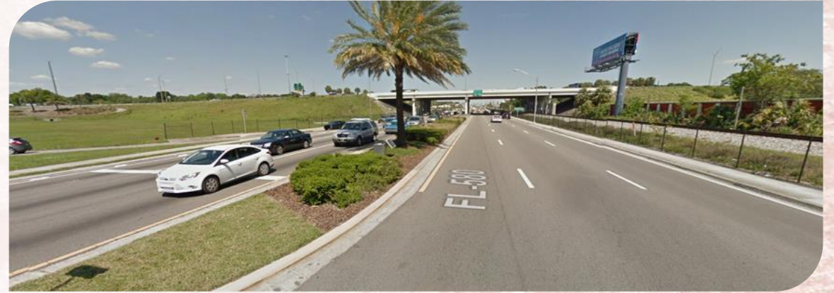
▲ Eastbound Busch Blvd. approaching I-275 Overpass
