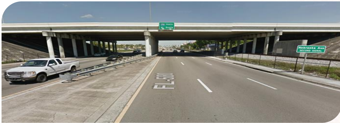
▲ Eastbound Busch Blvd. at I-275 Overpass
