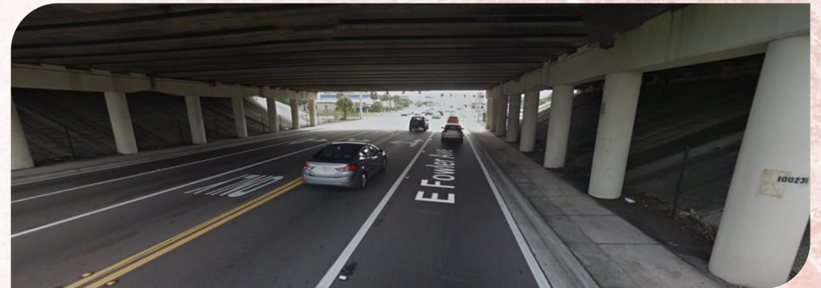
▲ Eastbound Fowler Ave. under I-275 Overpass
