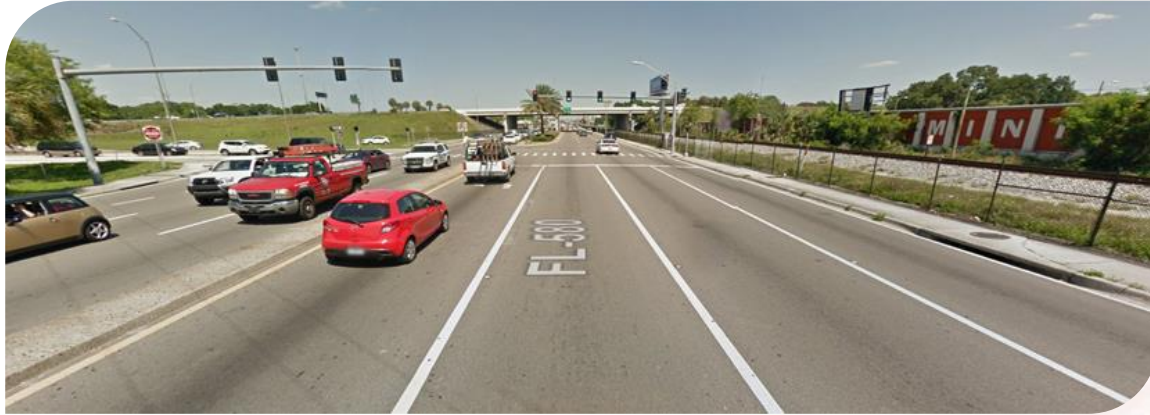
▲ Eastbound Busch Blvd. at Exit Ramp Intersection
