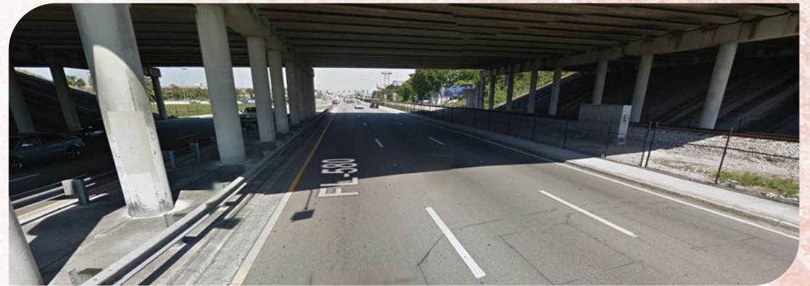
▲ Eastbound Busch Blvd. under I-275 Overpass
