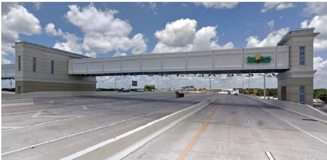
This toll gantry on the Crosstown Connector in Tampa spans the entire width of the roadway
