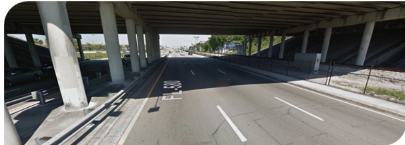
▲ Eastbound Busch Blvd. under I-275 Overpass
