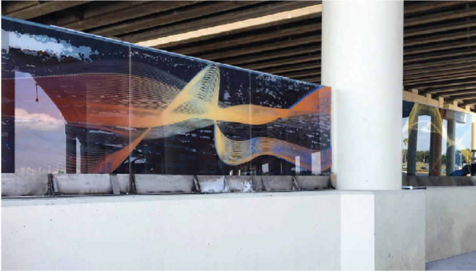
Art panels being installed along the Tampa Riverwalk
