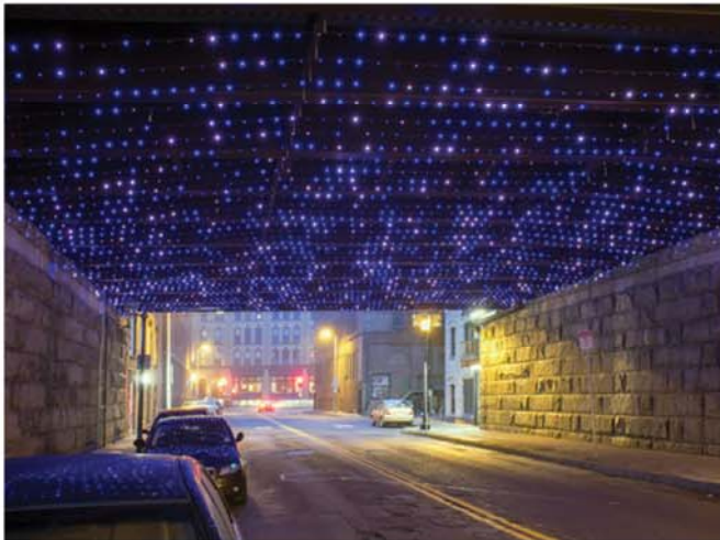
Under Bridge Lighting
