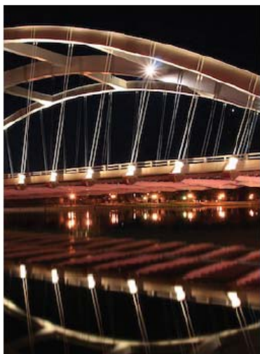
Bridgeway arch lighting
