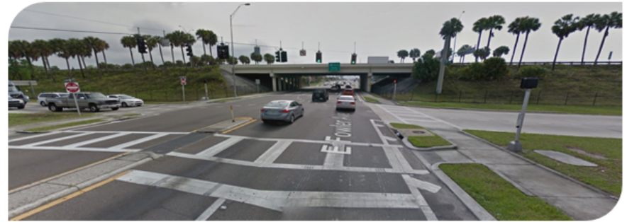
▲ Eastbound Fowler Ave. at Central Ave. Intersection
