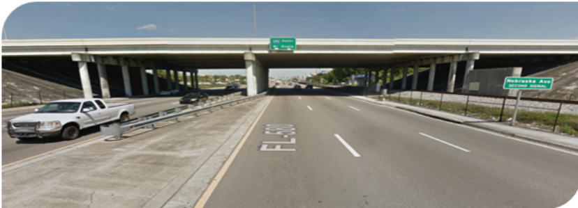
▲ Eastbound Busch Blvd. at I-275 Overpass
