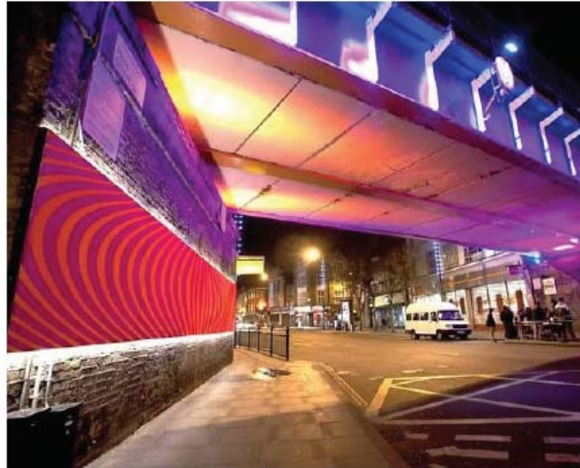
Underbridge lighting and aesthetics
