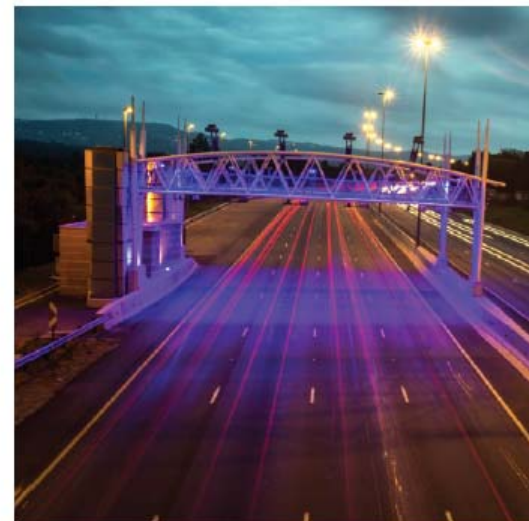
At night, this gantry creates a colorful aesthetic expression
