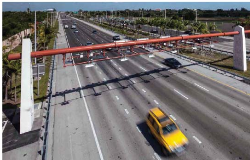
A painted monotube gantry with themed concrete piers on SR 836 west of Miami International Airport
