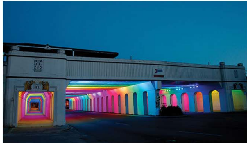
Under Bridge Lighting
