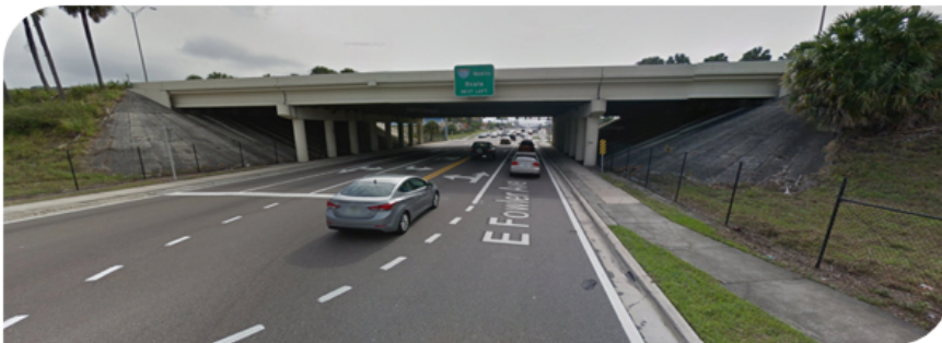
▲ Eastbound Fowler Ave. at I-275 Overpass
