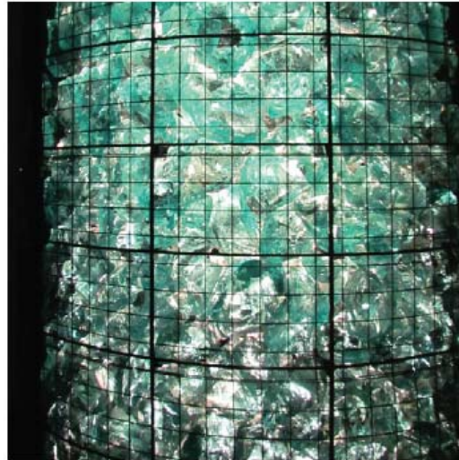
Recycled glass gabion
