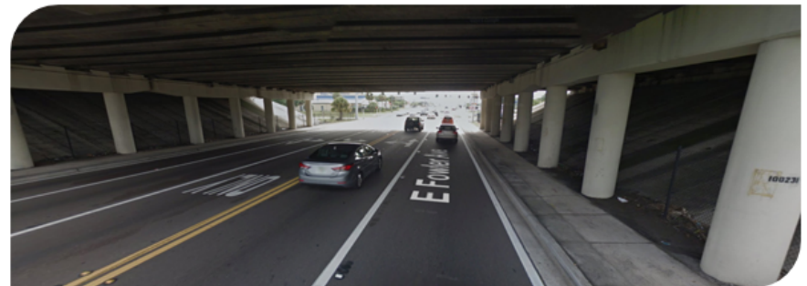
▲ Eastbound Fowler Ave. under I-275 Overpass
