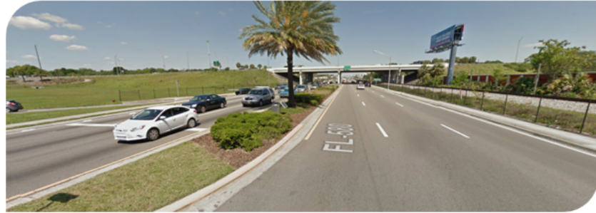
▲ Eastbound Busch Blvd. approaching I-275 Overpass
