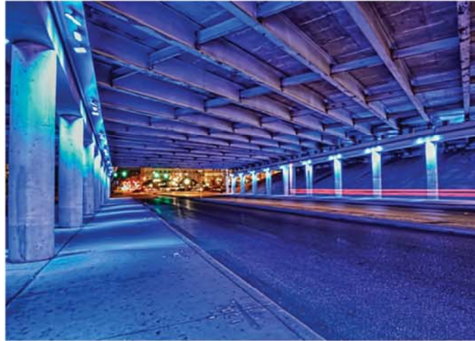
Under Bridge Lighting
