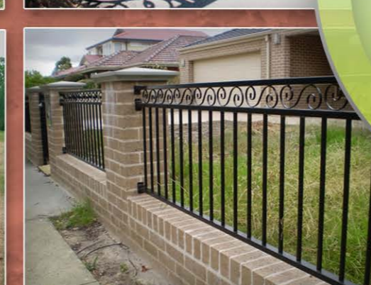
Combination masonry columns and iron pickets
