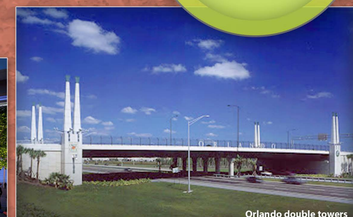
Orlando double towers
