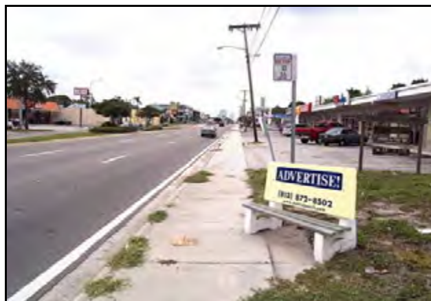
Figure 3-1 Examples of Sidewalk Condition
