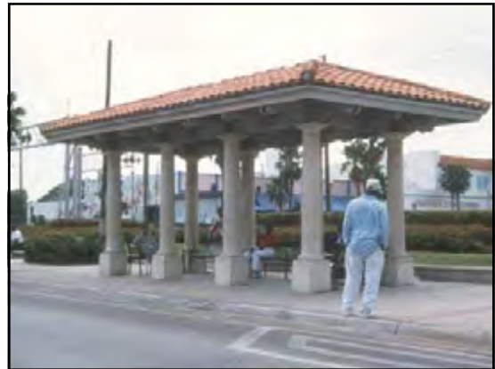
Figure 6-4 Examples of Transit Stops and Concrete Crosswalks
