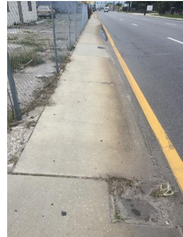
Florida Ave south of Lake Ave
