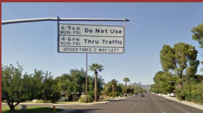
Arterial Roadway Reversible Lanes
