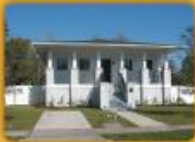
Aline Avenue Drainage Improvements
