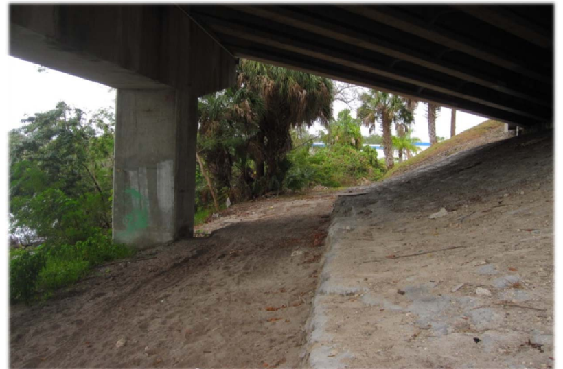
Underneath the Dr M. L. King Jr. Bridge, looking north
