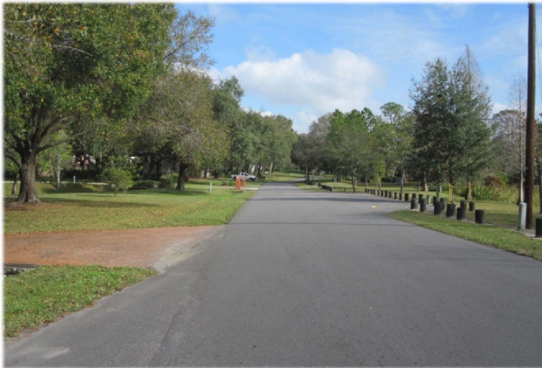
River Shore Drive, looking north
