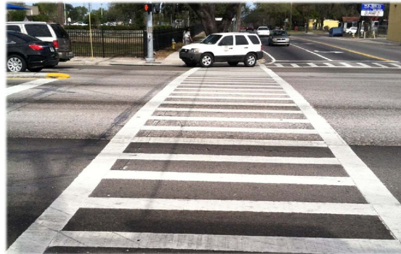
Figure 8: High Emphasis Crosswalk
