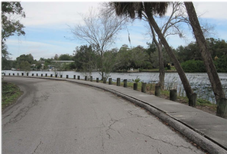
River Shore Drive, looking north
