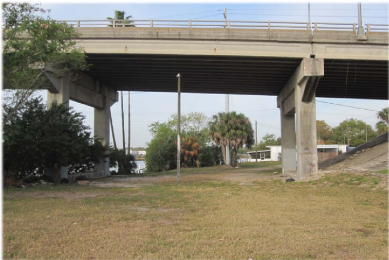
North Boulevard Bridge, looking west
