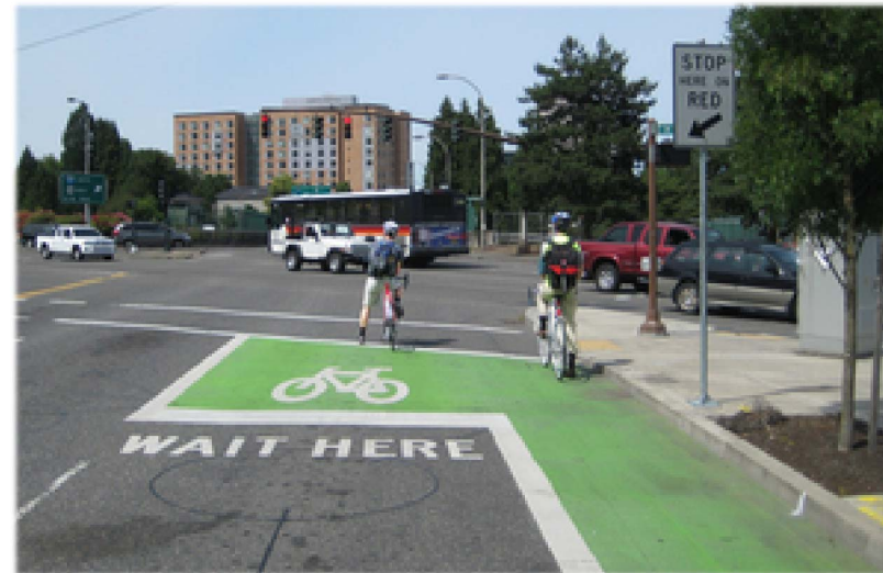
Figure 12: Bike Box at Signalized Intersection
