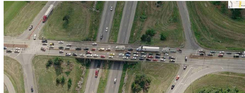
Figure 2.18: Rte 13/I-44 Interchange before Conversion
