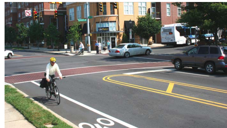
Figure 2.10: Complete Street, Charlotte, NC
