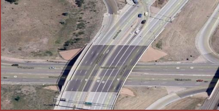
Arterial Roadway HOV Lanes
