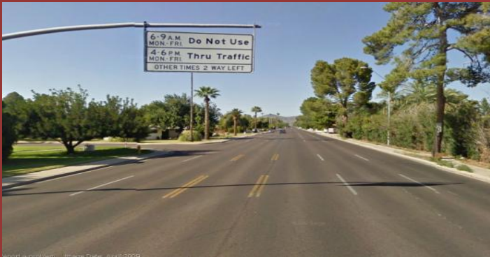
Arterial Roadway Reversible Lanes
