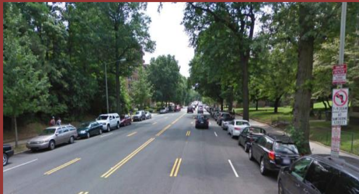
Arterial Roadway Time-of-Day Parking
