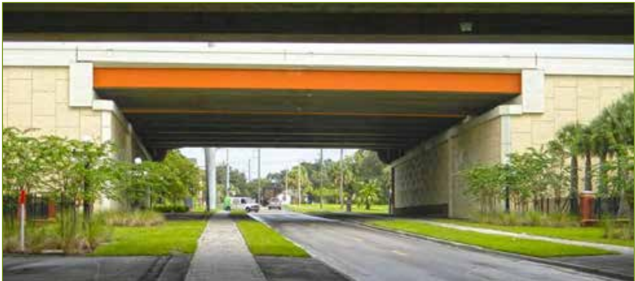
Figure 12: 26th Avenue at I-4 Overpasses
