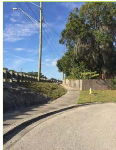
Figure 18: Existing 5-foot sidewalk at River Shore Drive and Hillsborough Avenue Bridge
