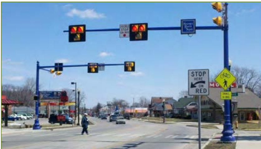
Figure 10: HAWK Pedestrian Crossing Signal with Trail Signage Source: nickelplatetrail.org; Fulton and Howard Counties, Indiana
