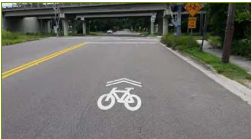
Figure 6: Shared Lane Markings – Euclid Avenue, Tampa
