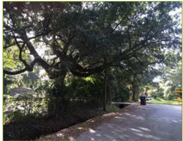
Figure 16: Drainage on Alicia Avenue
