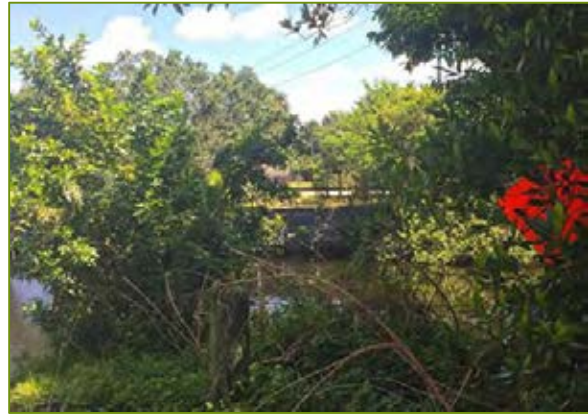
Figure 14: Extant remains of the streetcar/trolley crossing over the Hillsborough River on Van Dyke Place
