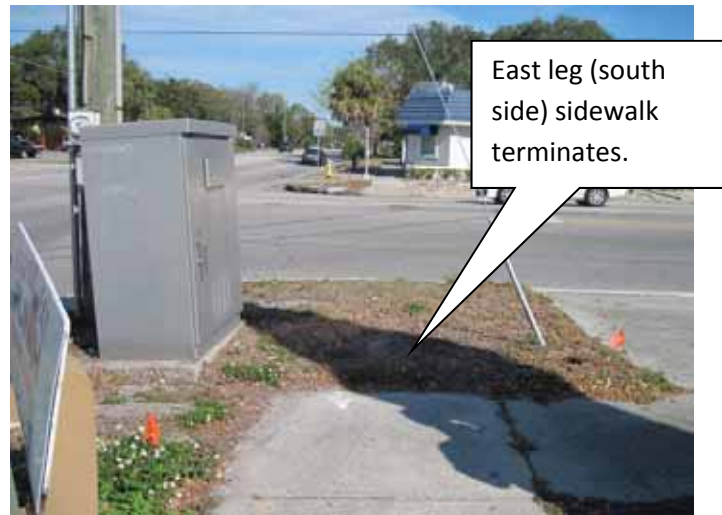
Figure 3C: Sidewalk gap crossing Bay to Bay Boulevard (looking north)
