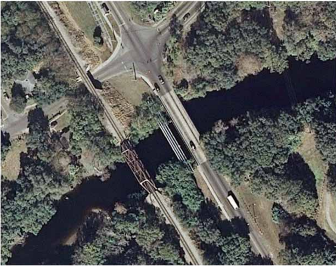
Figure 35B: Existing Rowlett Park Drive Bridge Aerial
