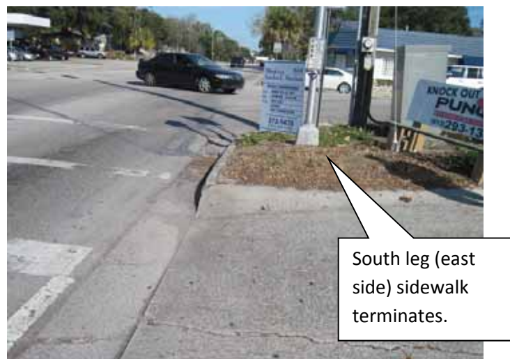
Figure 3D: Sidewalk gap crossing Manhattan Avenue (looking north)
