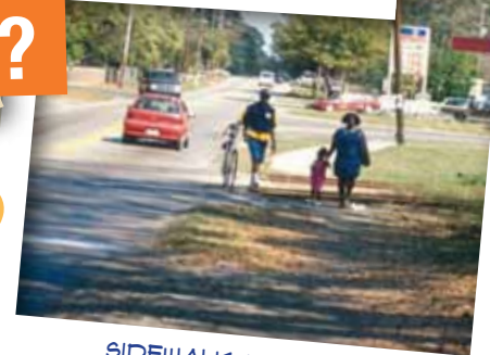
SIDEWALK REPAIRS AND INSTALLATION
