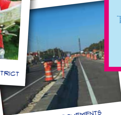
ROAD IMPROVEMENTS WITHIN THE DISTRICT
