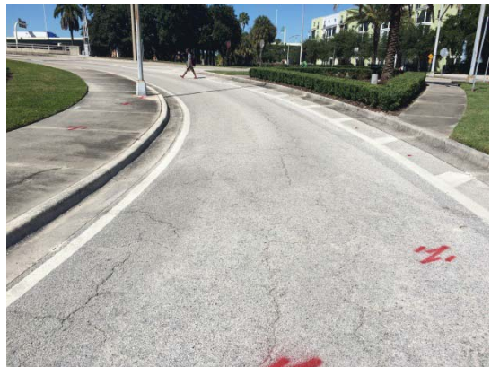
Right-turn slip lane, Laurel Street at Doyle Carlton Drive
