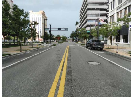
Zack Street between Tampa Street and Franklin Street, looking west
