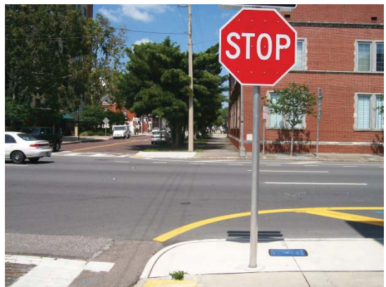
Harrison Street at Florida Avenue, looking east
