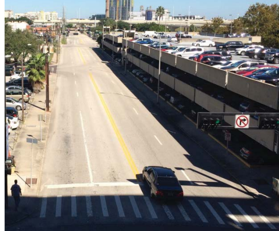
Whiting Street at Florida Avenue, looking east
