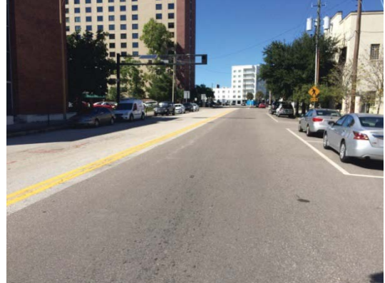
Marion Street at Tyler Street, looking north
