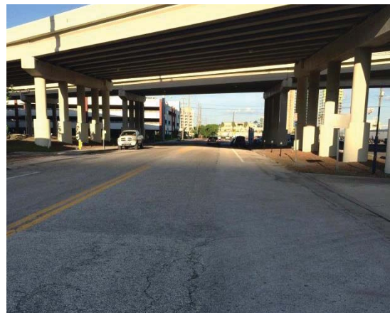
Whiting Street at Jefferson Street, looking east
