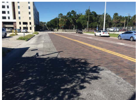
Morgan Street at Tyler Street, looking north
