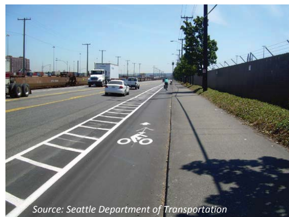
Source: Seattle Department of Transportation Figure 32: Example of a buffered bicycle lane
