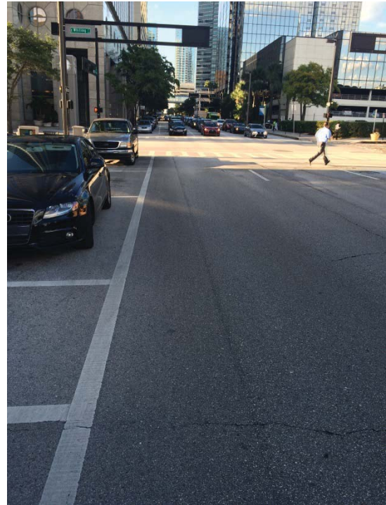
Tampa Street, south of Whiting Street looking north
