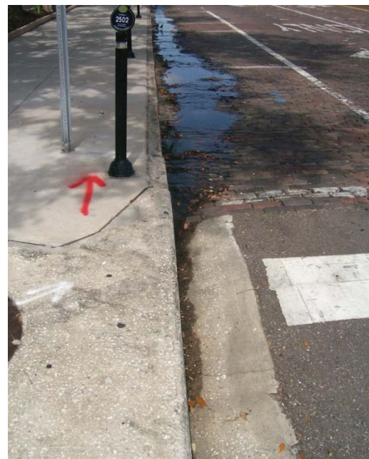
Drainage inlet and granite curbing along Twiggs Street
