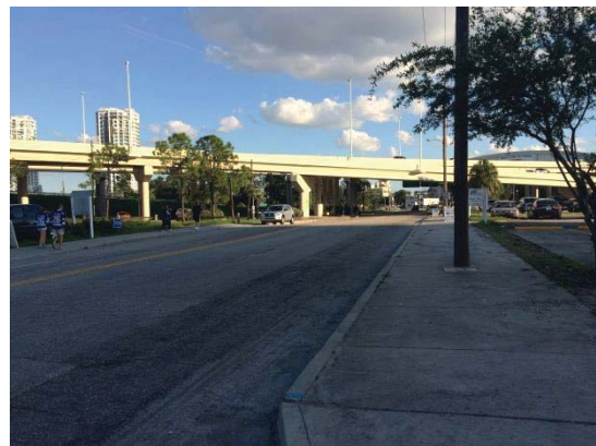
Jefferson Street at Whiting Street, looking south
