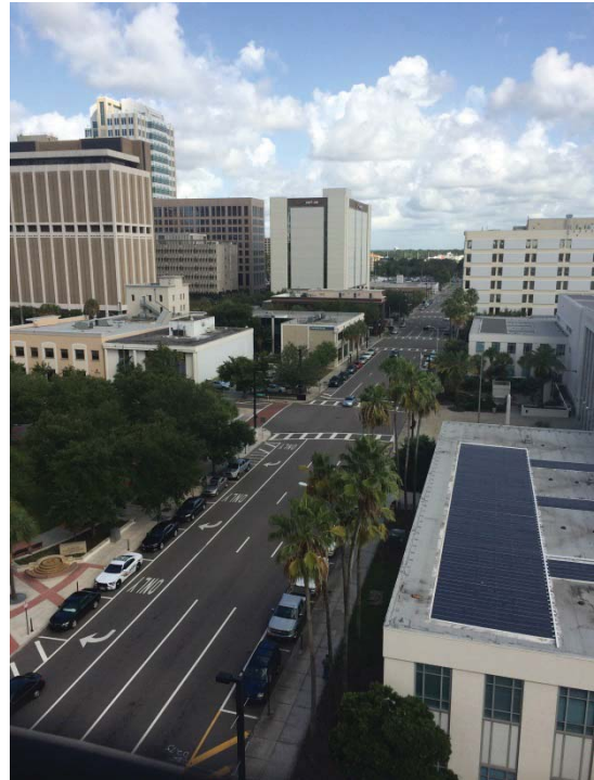
Pierce Street at Kennedy Boulevard, looking north
