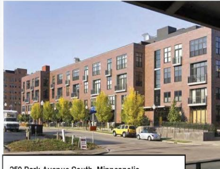
250 Park Avenue South, Minneapolis Adaptive Reuse Condominium project Near Downtown East/Metrodome Station Source: minneapolisloftsandcondos.com
