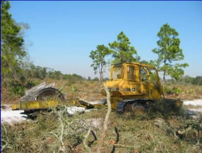
Dozer with Roller Chopper
