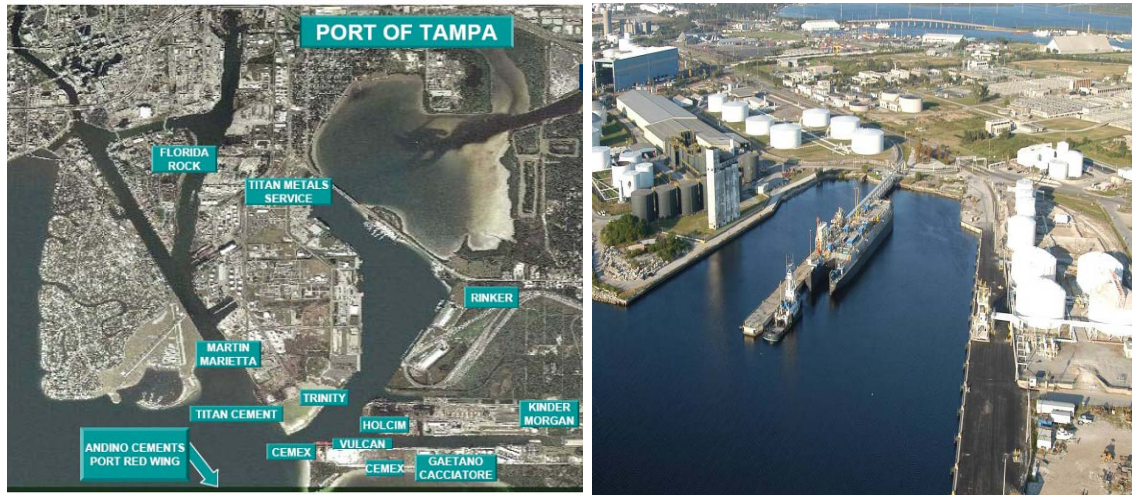
Figure 4: The Port of Tampa
