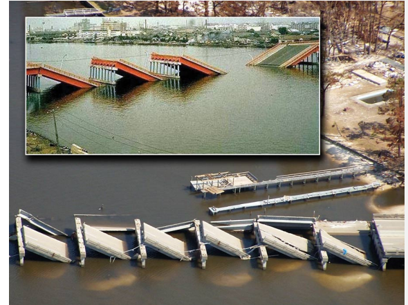
Impact of Hurricane Katrina to Bridges along the Gulf Coast Region
