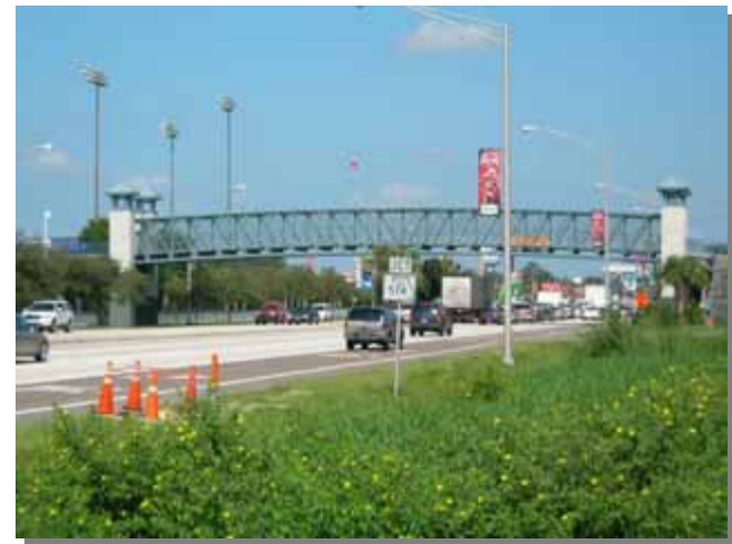
Figure 2.29: Pedestrians and bicycles are routed above this high volume road near Raymond James Stadium in Tampa
