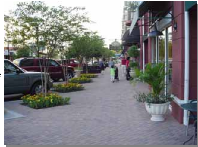
Figure 2.21: A wider sidewalk eliminates the need for passing areas
