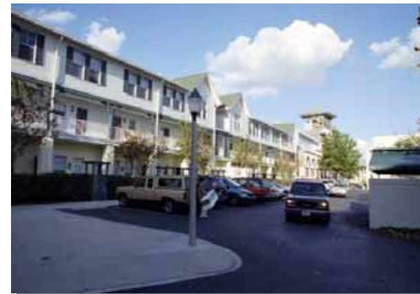
Figure 2.47: This rear parking area is accessed from side streets
