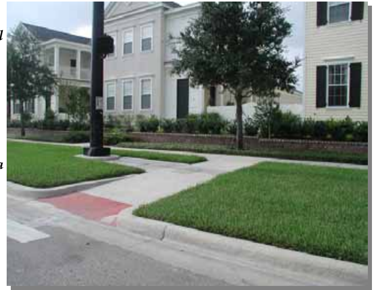
Figure 2.22: Typical tactile warning strip, its contrasting color and raised indentions warn pedestrians they are about to enter a vehicular zone
