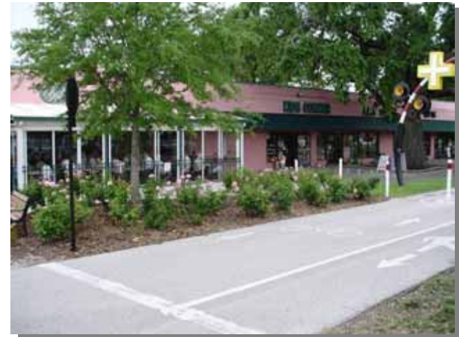
Figure 2.10: The markings on the pavement give directional information and separate bicyclists from pedestrians
