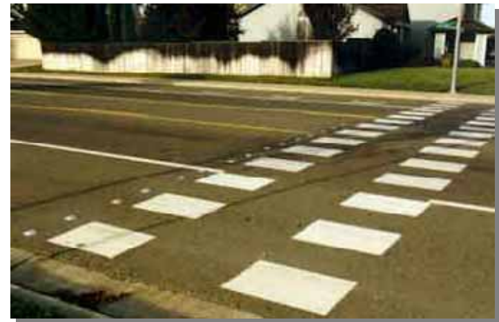
Figure 2.12: Triple-Four crosswalk markings
