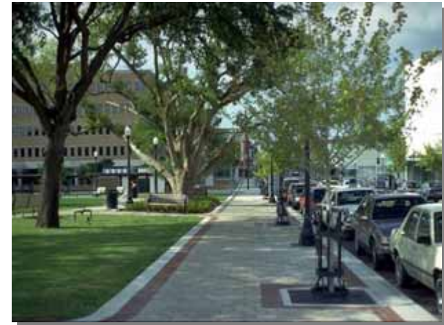
Figure 2.6: Sidewalk buffered from roadway by vehicular parking, pedestrian lighting, and landscaped areas. Although the clear passage width is the same as the above example, the sidewalk placement and buffers create a more pedestrian friendly environment
